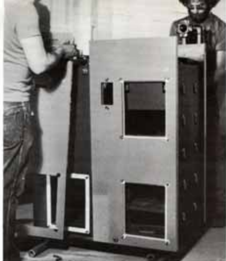
Installation of boiler jacket and mounting of doors and components can be done by homeowner to cut installation cost.
