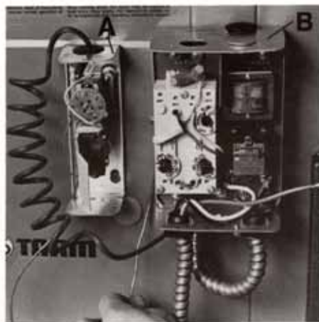
Connecting overheating control (A) and master hot-water control (B) normally requires skill of a professional.
