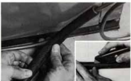
Oil feed line to burner was protected by slipping old garden hose (slit on one side; see inset) over the exposed tubing.
