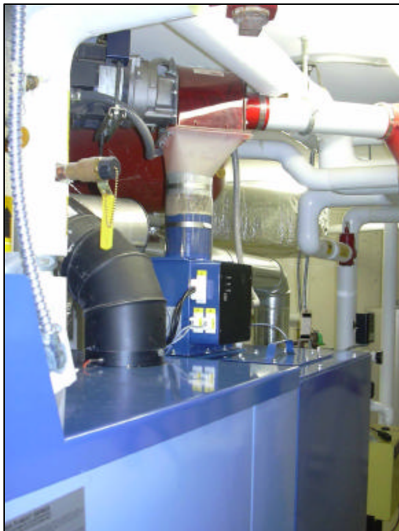
Side View Showing Automatic Feed Device and Auger
