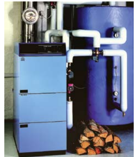
A heat storage system will produce and store hot water throughout the year.
