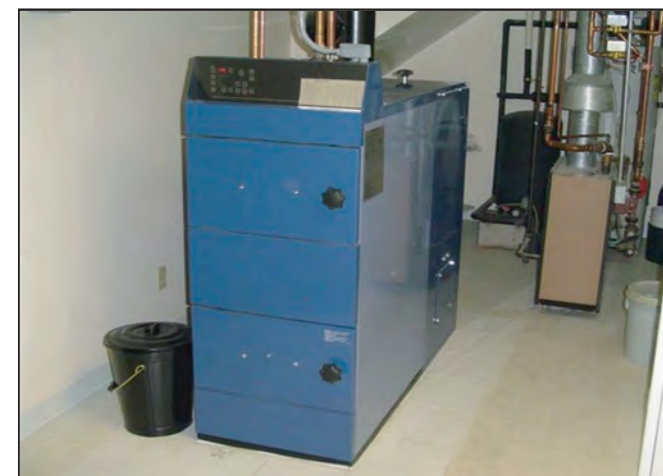
Multi-Heat: Fully automatic stoker boiler with hopper
